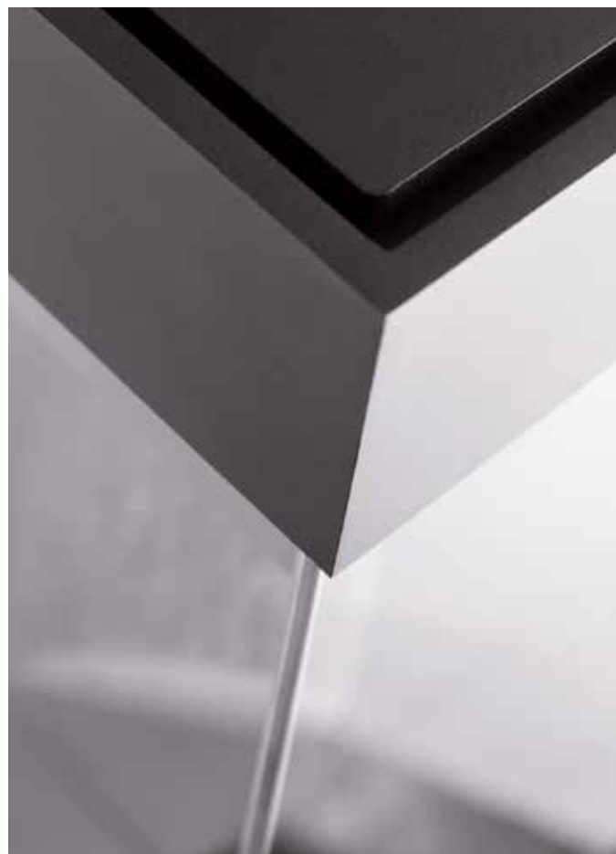
Glass-to-glass without corner profile
